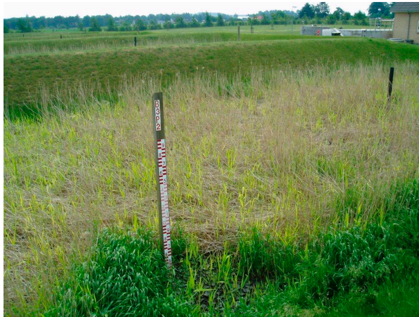
Figure 5. Yellow reeds and poor coverage in an STRB (Stenlille, Denmark) loaded with sludge rich in nickel (courtesy of Orbicon).
