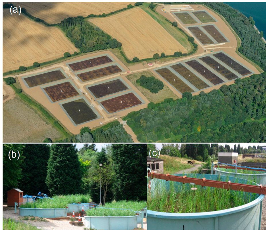
Figure 8. (a) Full-scale and (b,c) pilot-scale STRB systems [38,59] at Hanningfield (England) for water works sludge dewatering (courtesy of Orbicon).
